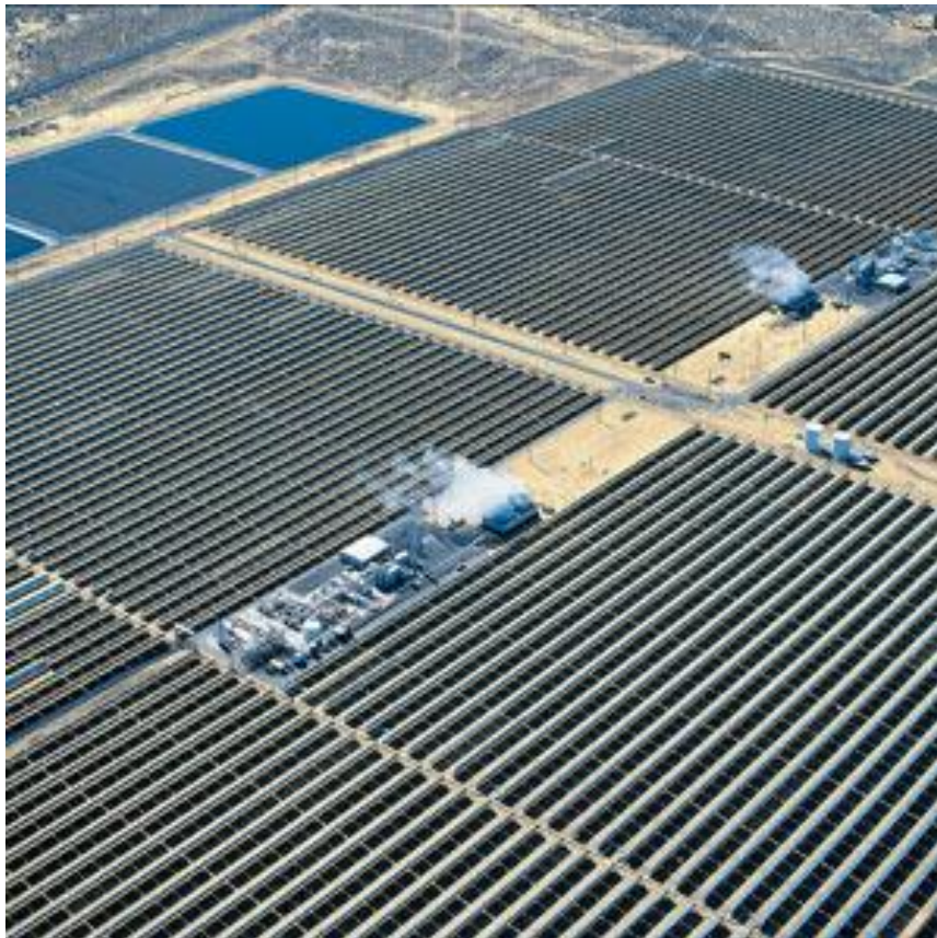
Image 3.7: Solar Power Plant
