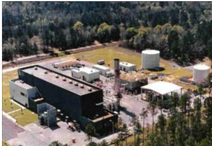
Image 3.30: Compressed Air Plant
