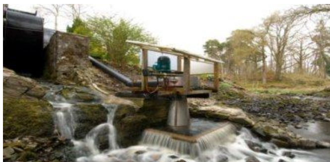
Image 3.16: Small-Scale Hydroelectricity Facility
