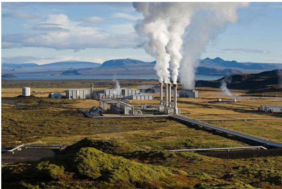
Image 3.15: Geothermal Power Plant
