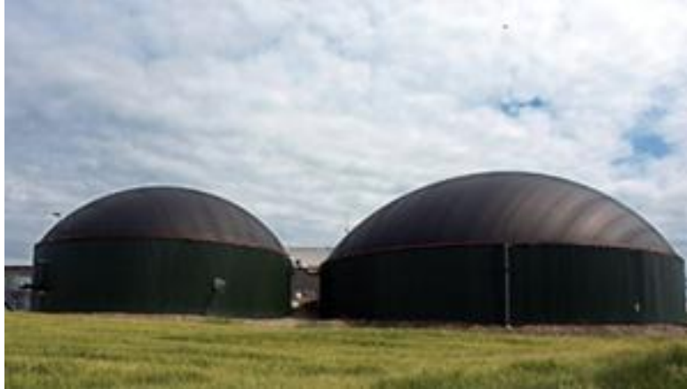
Image 3.13: Biogas Power Station
